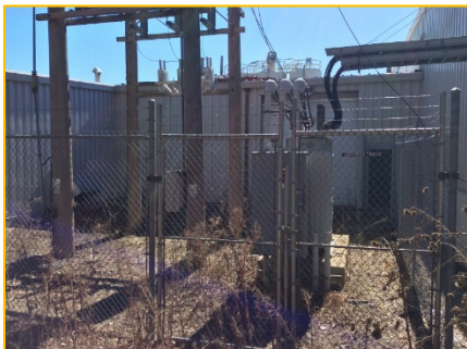
The undocumented PCB content of an onsite electrical transformer was listed as a REC for the subject property.
